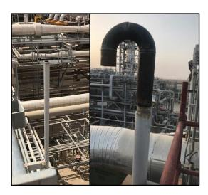
**Figure 8:** Dry gas seal secondary seal leakage vent line before and after modification.
