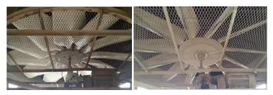
Figure 2 Before & after upgrade to fiber plastic
