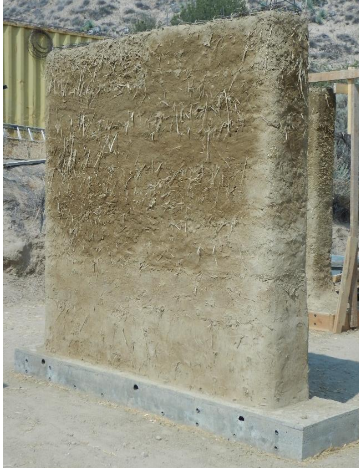
Figure 6.7: Pipe Stem Wall before Testing
