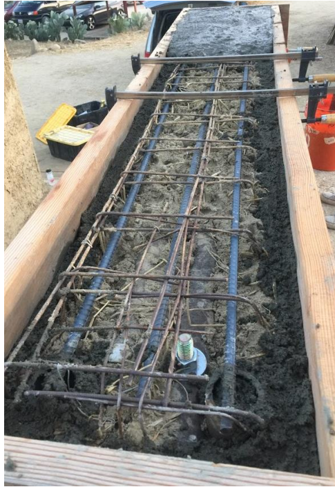
Figure 4.5: Concrete Reinforcement
