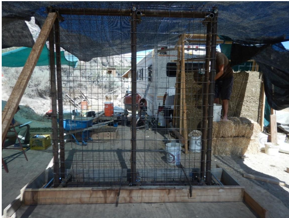
Figure 4.3: Complete Reinforcement in Foundation Form
