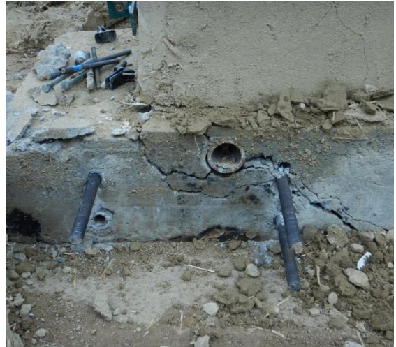
Figure 6.11: Foundation at Failure
