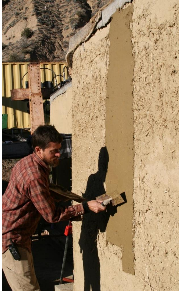
Figure 6.5: Thin Plaster Layer Applied to Wall
