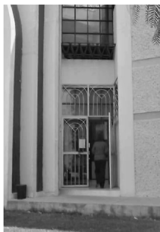
Photograph 6: The entrance to the SAC building
