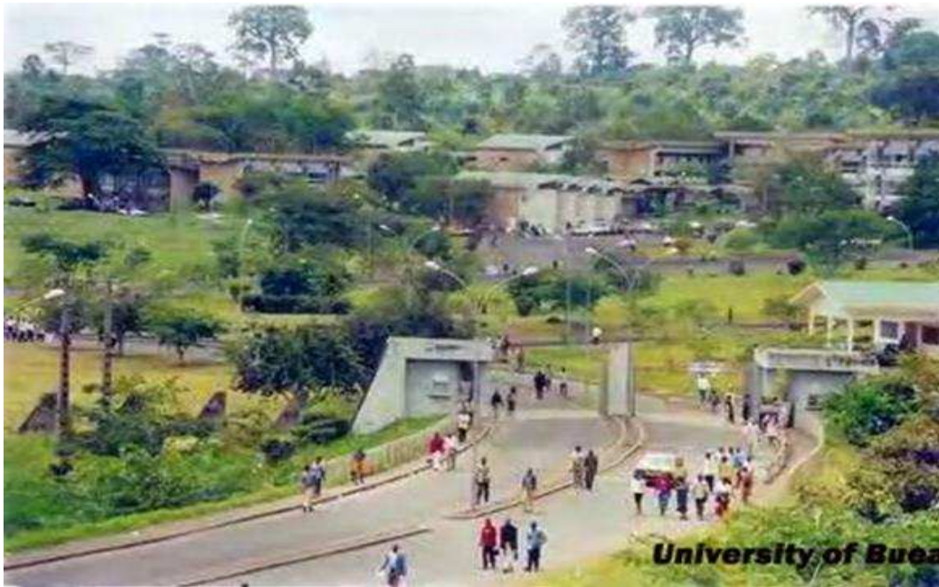
Figure 3.3: A sectional view of the University of Buea.
