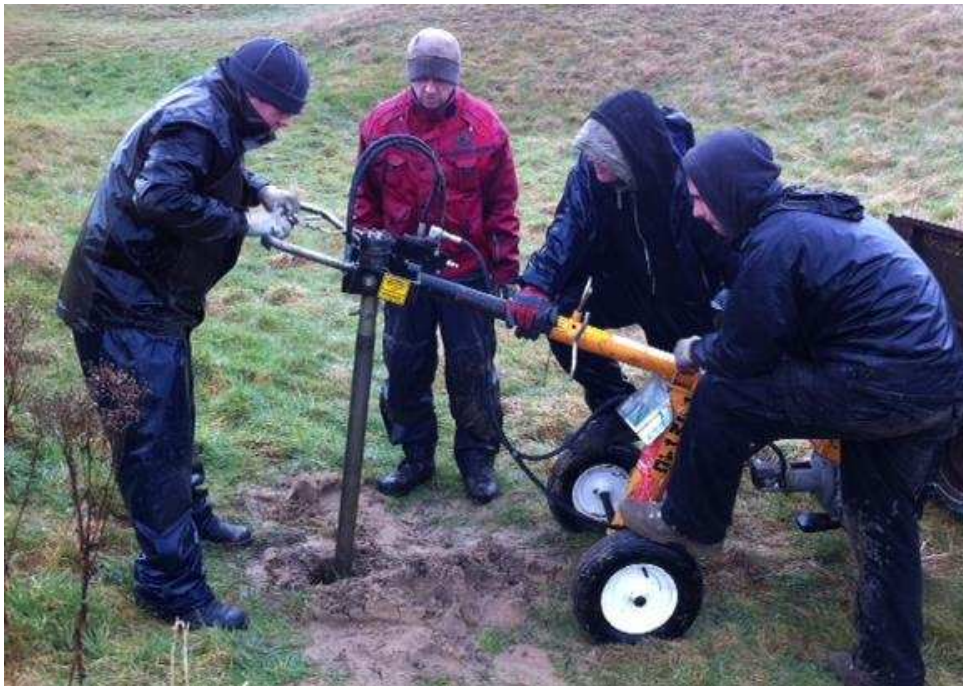
Plate 3.1 Dipwell installation using the two-man hydraulic auger
