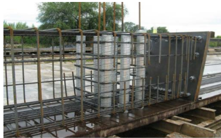
Figure 2.11. Pretensioned precast cap (Miller et al., 2014).
