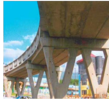
(b) Underside of the Completed Bridge
