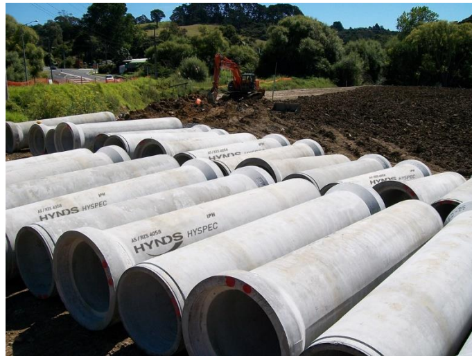
Figure 3. Rubber Ring Jointed Drainage Pipe
