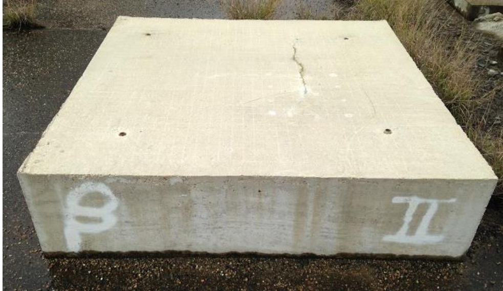
Figure 5.1: Hollow Rods Shown in the Four Corners of Slab II
