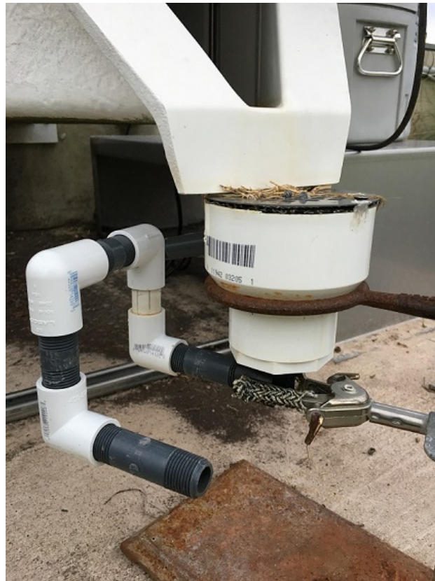
Figure 3.1: Second-generation runoff sensor installed in the turfgrass field laboratory for field-testing.
