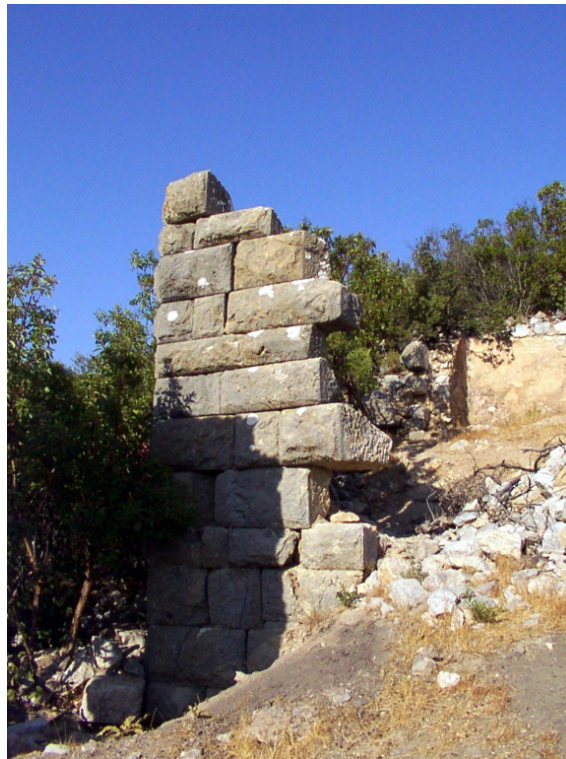
Figure 6: Surviving tower constructed of rusticated ashlar masonry at Lamos
