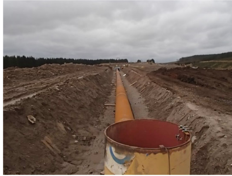
Fig. 1. Image of the test section prior to being backfilled.
