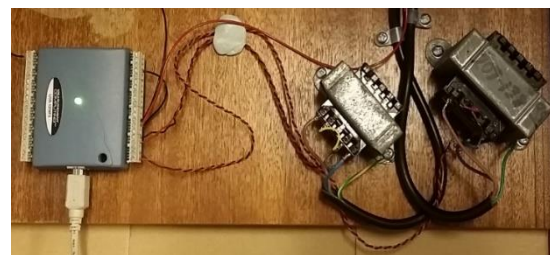
Figure 3.23. Illustrate the setup used to measure, digitize and record mains signal directly through
