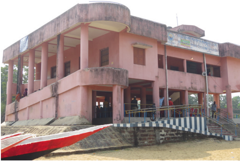
Fig. 11.1 Effective local adaptation infrastructure: Cyclone shelter in the Mahanadi Delta, India (Photo: Amit Ghosh/Shouvik Das)
