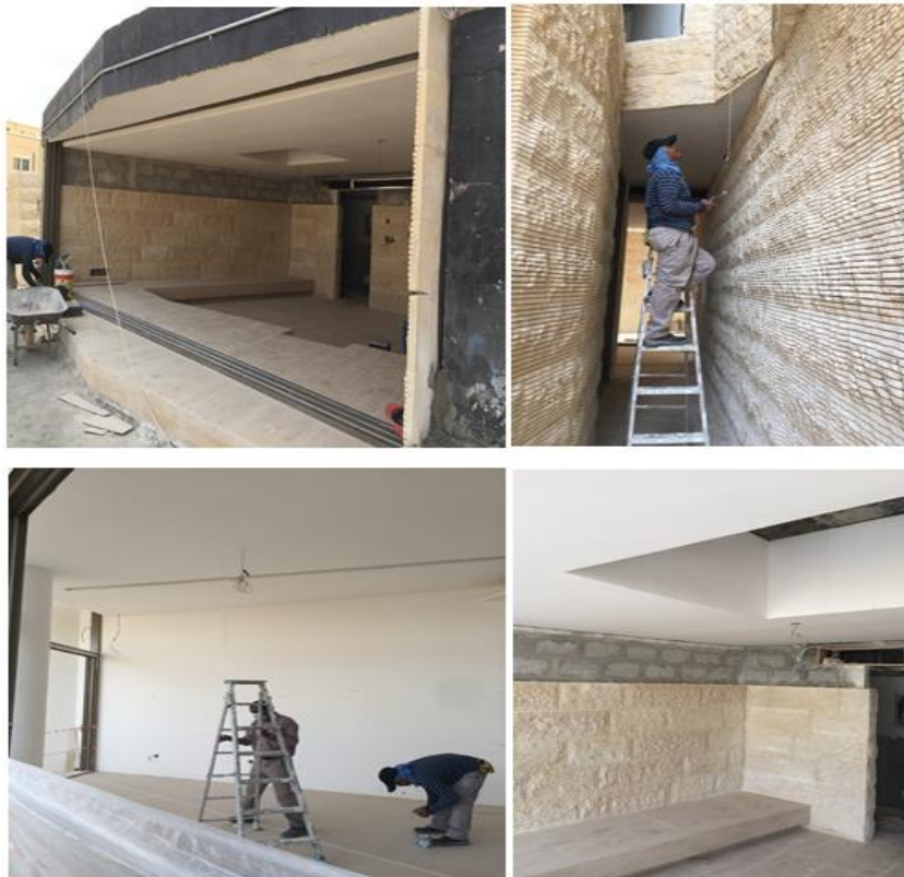
Figure 89: Site visit January, 2016 – Site remain under-construction – the chosen spaces.
