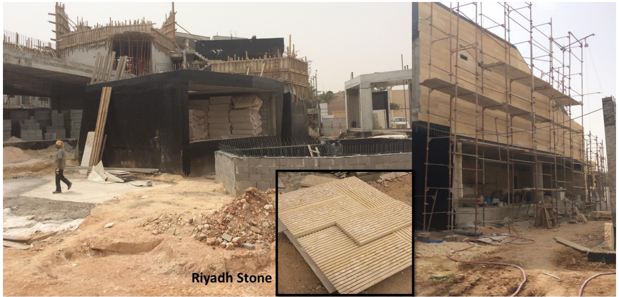
Figure 87: Site visit January, 2015.
