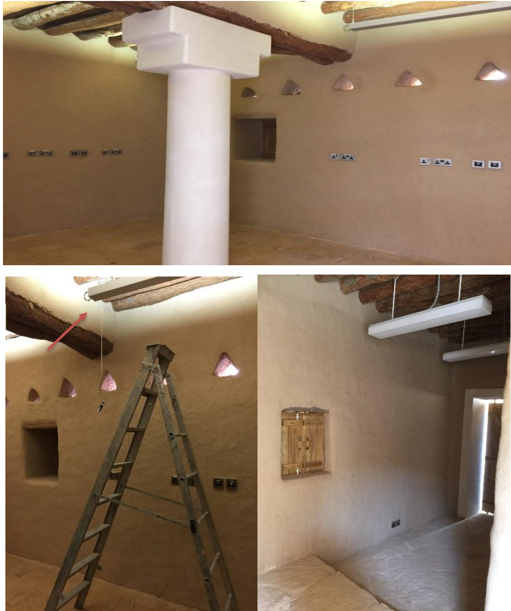
Figure 70: Addiriyah 2nd Indoor space – from July till December 2016.
