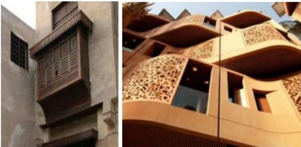
Figure 1: Traditional and Modern Mashrabiya in Middle East (Source: Ajaj and Pugnloni, 2014, p.228)
