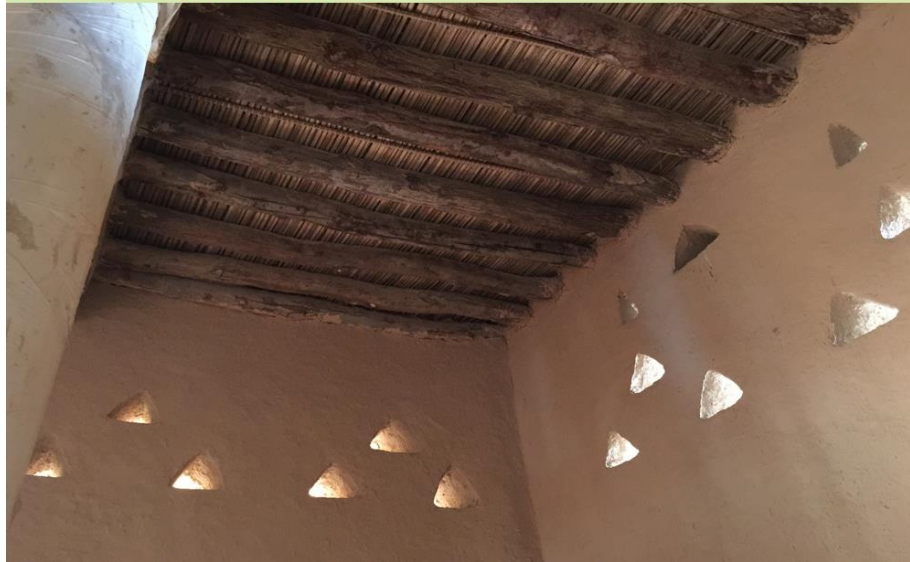
Figure 68: Addiriyah Indoor space.
