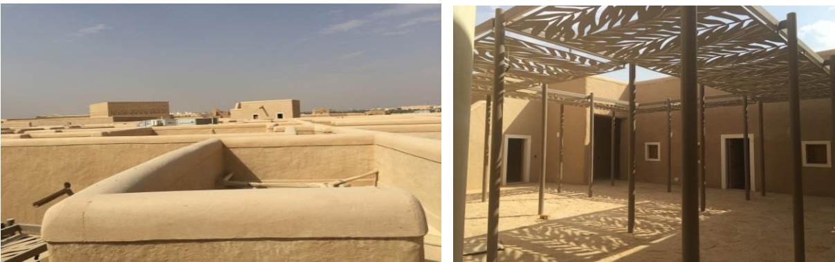
Figure 63: First site visit photos from January 2016, roof and courtyard
