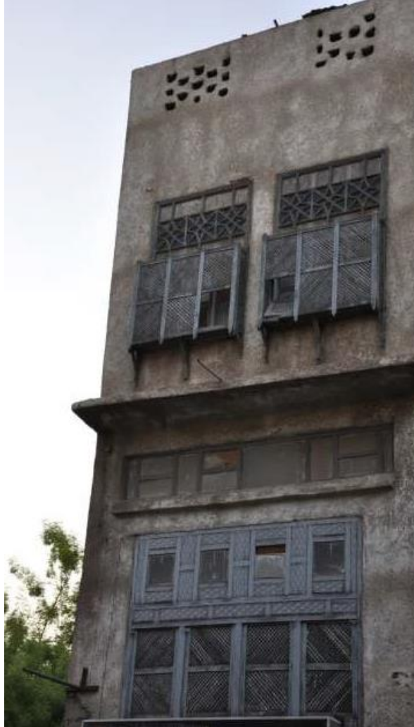
Figure 113: Traditional building in the Al Madinah city
