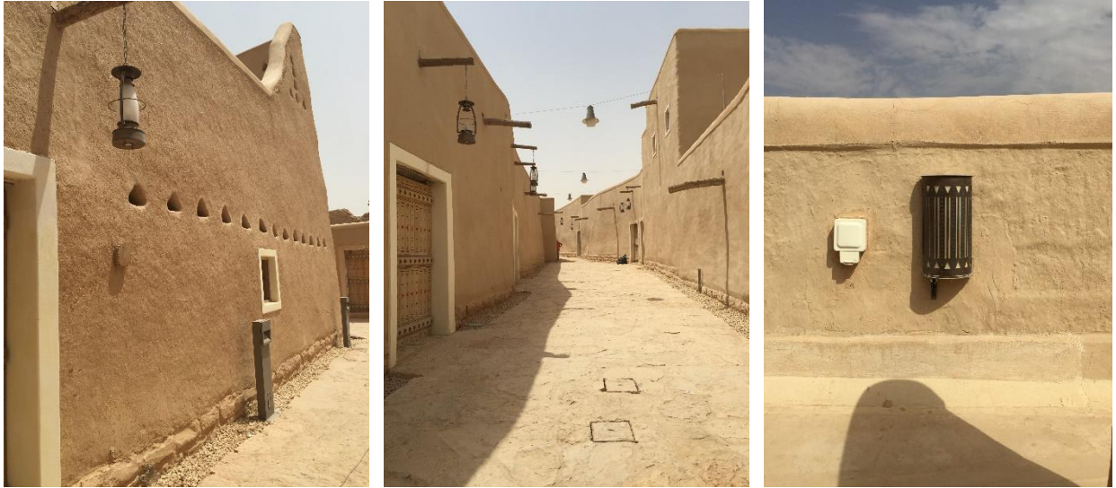
Figure 80: Addiriyah 1st Outdoor space – from January till March 2016
