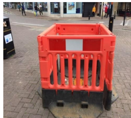
Picture 6: Further repair works
