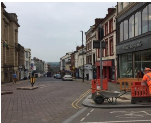
Picture 5: Repair works
