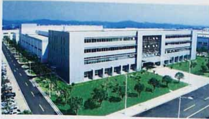
Figure 23 - CSR Times power electronics production base
