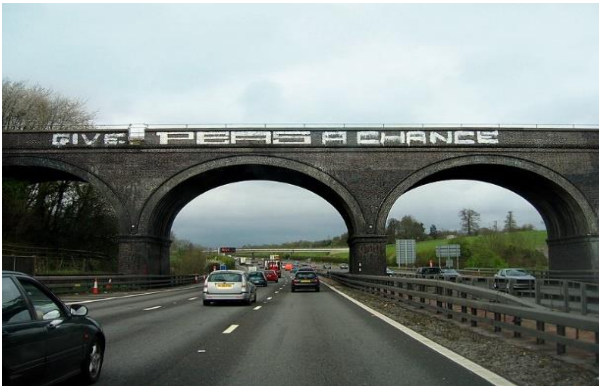
Figure 41: The Chalfort viaduct at Gerrards Cross, known as the 'give peas a chance bridge' crossing the M25 in England with its famous graffiti 'GIVE PEAS A CHANCE'. Sebastian Ballard under the Creative Commons Attribution-Share Alike 2.0 Generic.
