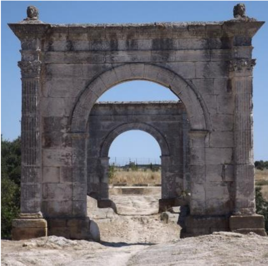
Figure 48 & 49: The Pont Flavien in Saint-Chamas in France, one of the few Roman bridges to retain both its original arches. An inscription can just be made out just above the arch. Author images.
