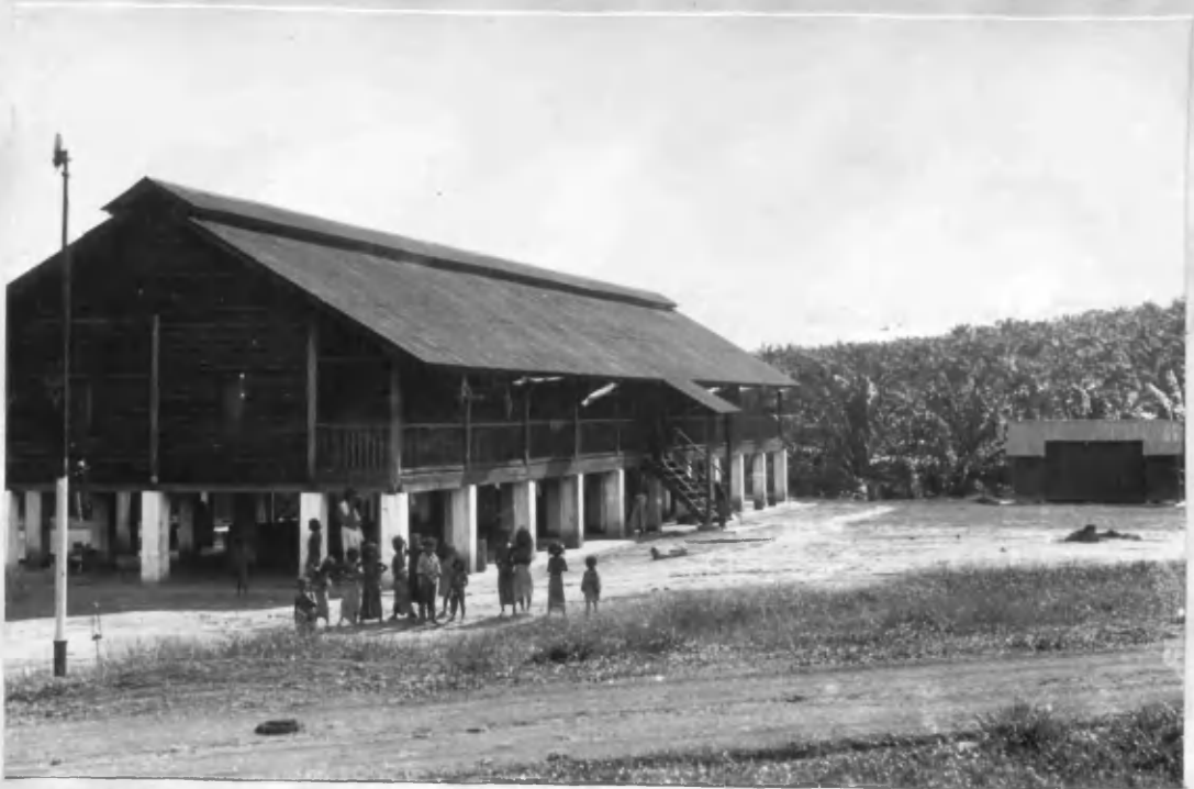
COOLY LINE. ESTATE "A" Shewing latrine on right. Oil palms beyond.
