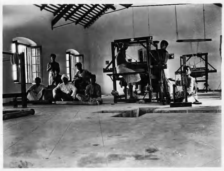
17. Interior View of the Industrial Sheds.
