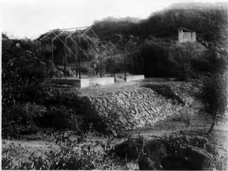
12. The Framework of the Infectious Diseases Hospital. Easily assembled when it was desired to employ the hospital, the covering was of thatch. See p. 26.
