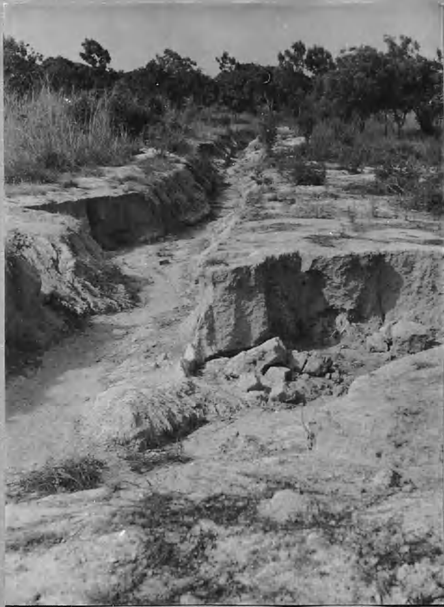
GOLD COAST. The effect of three inches of rain on one day on a well cut drain.
