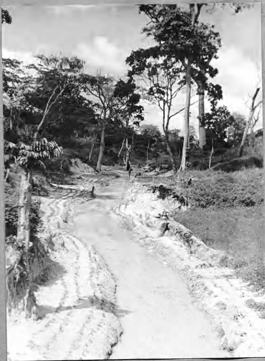
KINTAMPO. Canalisation of a stream and grass planting of the banks. In tsetse fly country.
