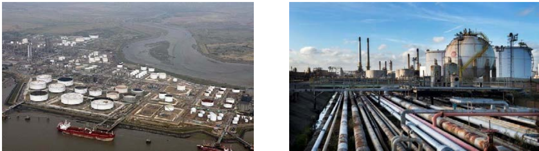
Fig. 1. (a) Coryton Oil Refinery as a working industry; (b) Same site after closure.
