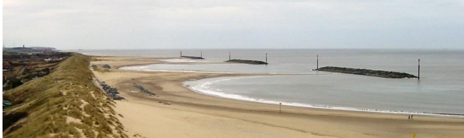
Figure 7. Beach response to detached breakwaters at Sea Palling, UK. Accretion of the shoreline toward the structure can be observed.
