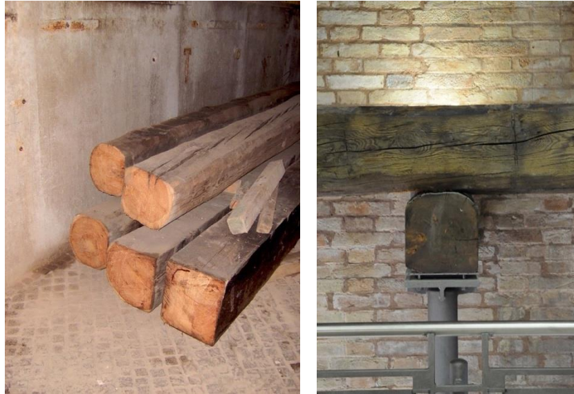
Fig. 2 – Reuse of old larch beams and cast-iron columns in an adaptive reuse project in Venice.
