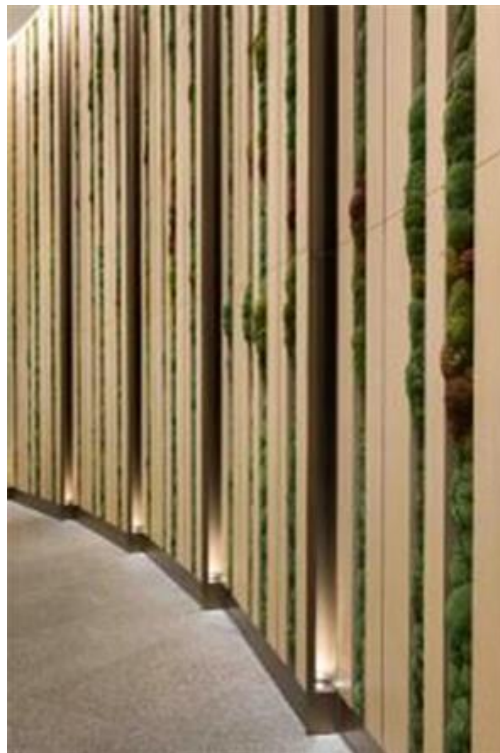
Figure 2-9: Creating sequences in the space by using lines in the wall curve. Source: Yu, Bai and Wu (2018).
