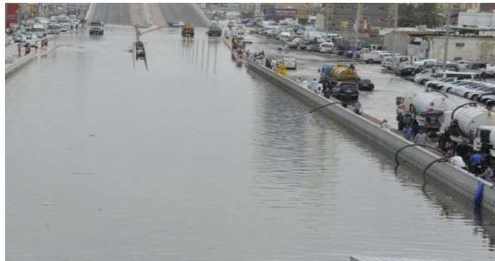
Figure 3-8: Using generators to suction the rainwater. Source: Al-Fahmi (2017).
