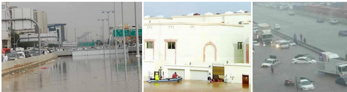
Figure 3-7: Sequential images about the damage that occurred due to the rainfall in 2009, 2010 and 2017 in Jeddah. Source Left to right: Al-Omair (2009); Al-Zahrani (2010); Sulaiman (2017).
