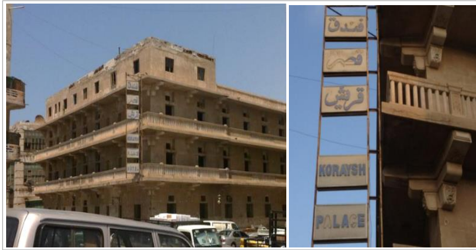
Figure 3-12: Images of Quraysh Palace Hotel in Jeddah. Source: Arfaj1 (2012) and Qdem (2012).
