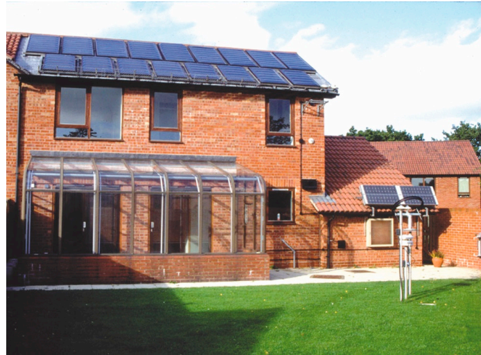
Figure 6. Solar Demonstration House in Bournville, Birmingham (see [3]).
