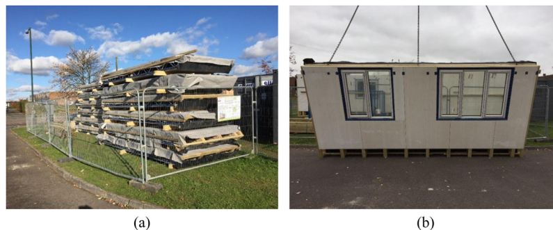
Fig. 7. (a) Prefabricated panels delivered to site (b) with pre-installed windows.
