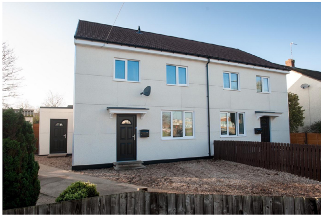
Fig. 9. A photo of the completed retrofit (source [7]).
