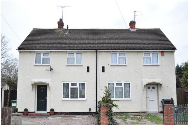
Fig. 1. Houses to be retrofitted.
