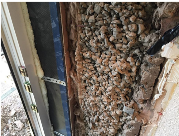
Fig. 2. Solid concrete in the external wall revealed during the retrofit process.
