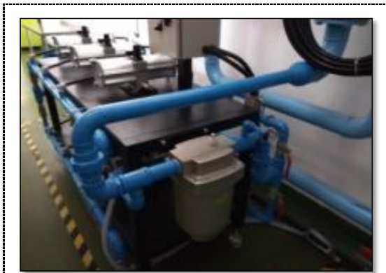
Figure 5. Booster pump installation along the compressed air line.
