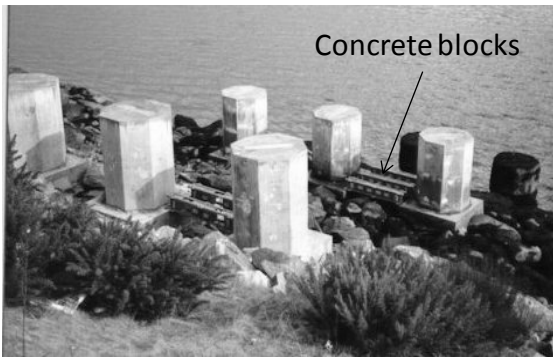
Figure 7. Concrete pier stems and concrete blocks exposed to different exposure classes
