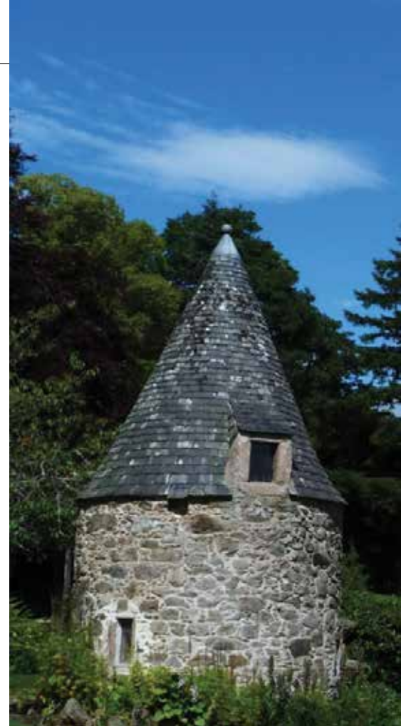
▲ Replacing cement render with replica feebly hydraulic hot-mix lime harling and lime wash at 17th-century Craigievar Castle, Alford, Aberdeenshire
