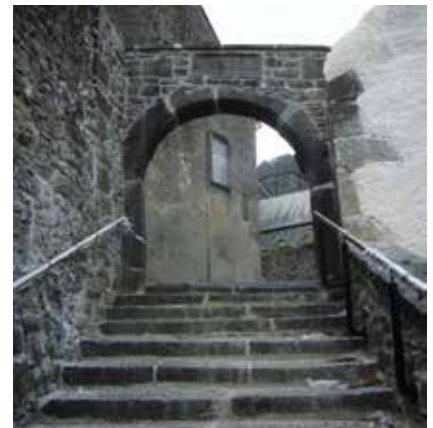
▲ 17th-century St Canice's Steps and Arch, Kilkenny, where masonry repairs and repointing of used feebly hydraulic hot-mix mortars
