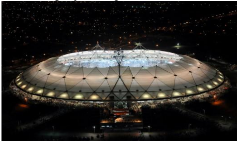
Figure 3. Roof of the stadium "La Plata Stadium" in Argentina.
