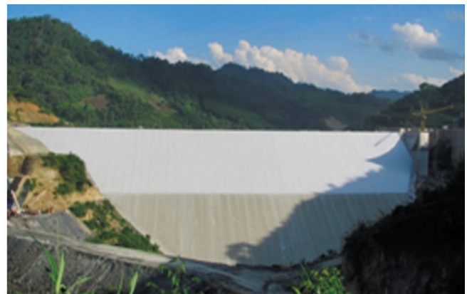
Fig.3. Nam OU VI rockfill dam after completion of the second stage installation of the exposed SIBELON® geomembrane system
