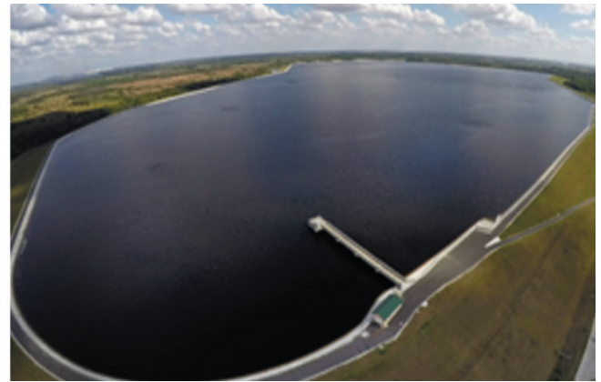
Fig.5. C.W. Bill Young reservoir in operation after rehabilitation, which included placement of a covered SIBELON® geomembrane system
