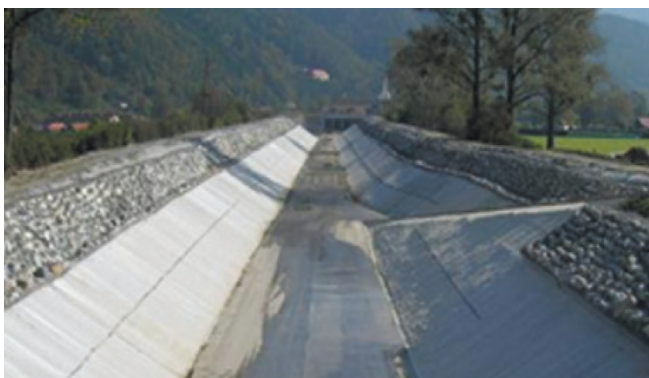
Fig.7. Pernegg canal after completion of the waterproofing works
