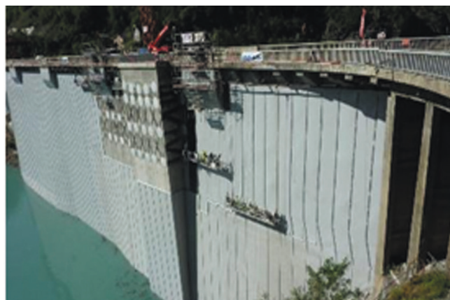
Fig.1. Installation of the SIBELON® geomembrane system at Chambon dam
