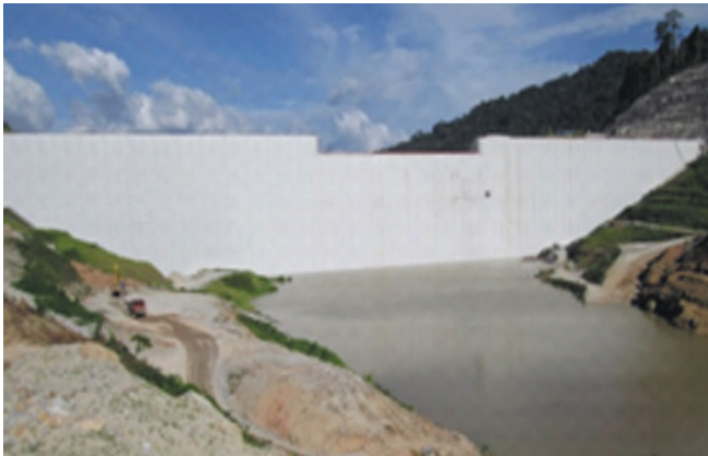
Fig.2. View of Susu dam during impoundment
