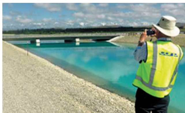
Fig.8. Tekapo canal after completion of the remedial works
