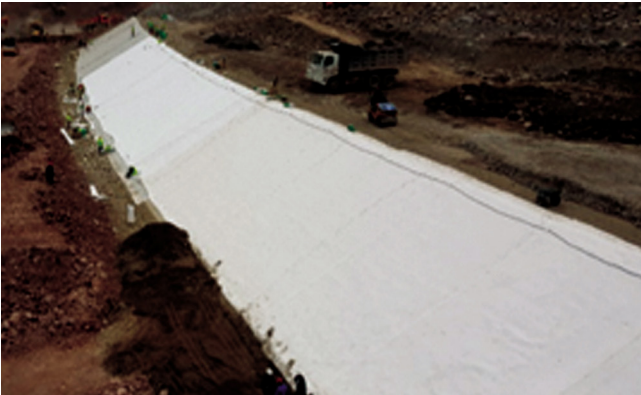
Fig.4. Installation of the SIBELON® geomembrane system in the Rogun upstream cofferdam
