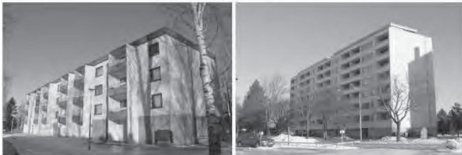
Figure 5 Typical Finnish suburban precast concrete buildings.
