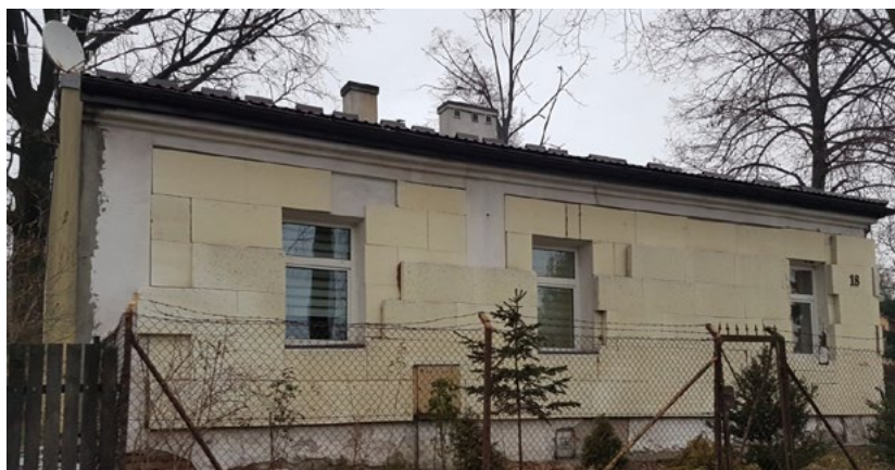
Fig. 1. An attempt to insulate the building from the outside, photo. K. Janus
