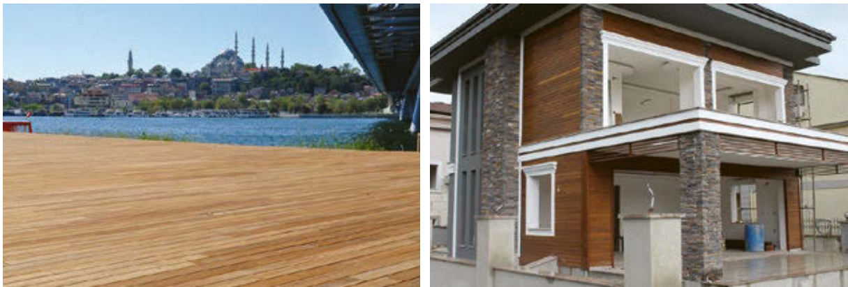
Figure 44: Examples of the use of modified wood: thermally modified wood decking (left), and thermally modified iroko wood cladding (right)
