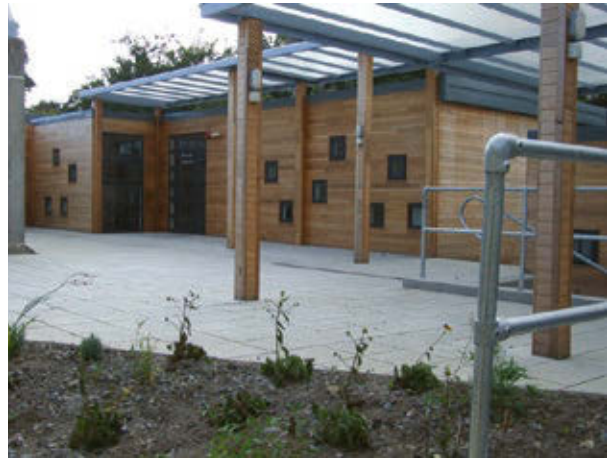
Figure 26: Example of Accoya board (left), and ThermoWood cladding on St Andrews College, Dublin (right)
