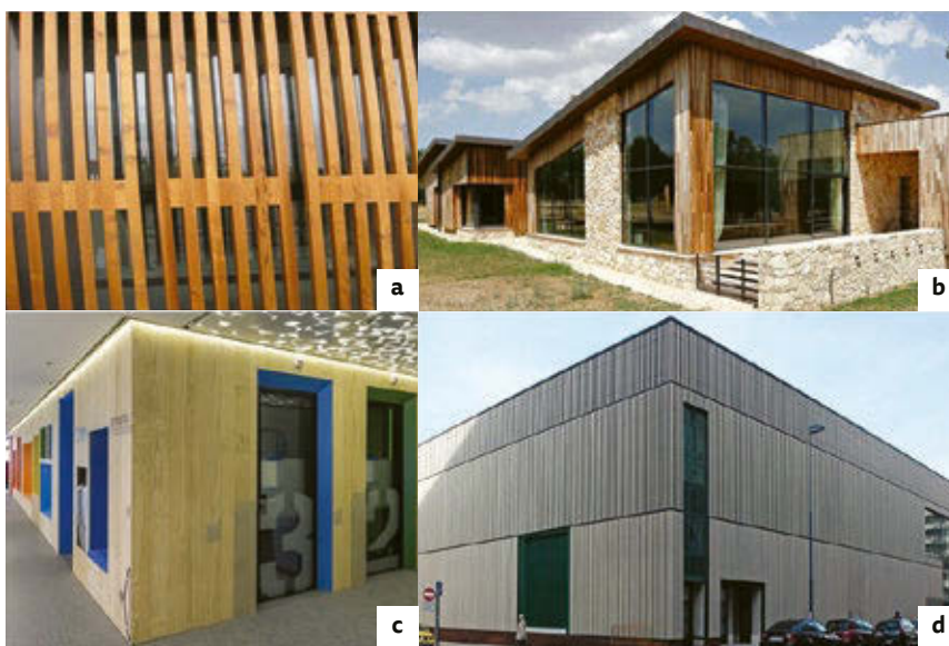
Figure 40: Examples of the use of modified wood: a) Façade of thermally modified Radiata pine, Madrid, b) façade of thermally modified Eucalyptus, Segovia, c) Accoya interior panels, Google office Madrid, and d) Accoya façade, congress palace Vitoria
