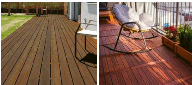
Figure 36. Thermally modified pine for decking from http://www.pardoseli-lemn.ro/deck/autohton/pin-termotratat/ (left), and thermally modified ash for decking and flooring from https://decolandia.ro/terase-din-lemn-si-pardoseli-exterioare/podele-terasa-decking--frasin-thermo (right)
