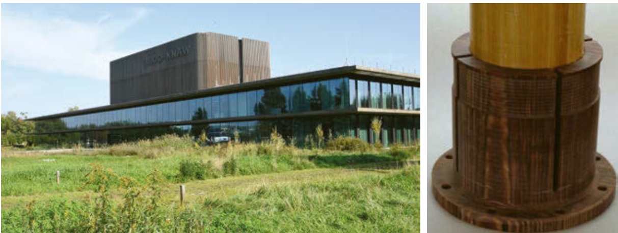
Figure 30: Plato thermally modified wood cladding (left), and fitting of densified resin-impregnated and laminated beech veneer (Dehonit®) from Deutsche Holzveredelung Schmeing GmbH & Co. KG (right)
