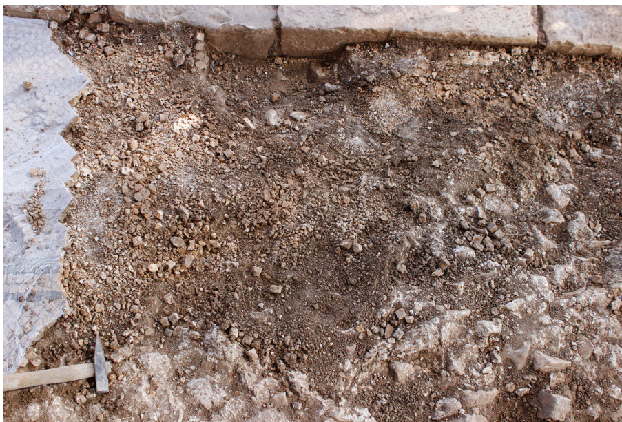
FIG. 8. Remains of the bedding and soil layer after lifting a mosaic section in Room 3.
