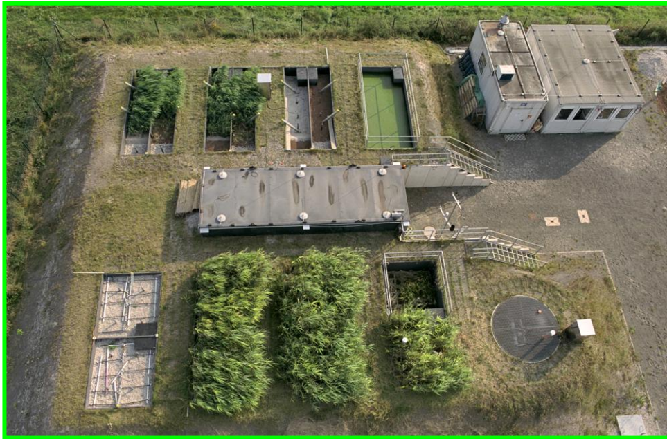
Photo 1.1: Bird eye view for the pilot plant in Langenreichenbach, Saxony, Germany.
