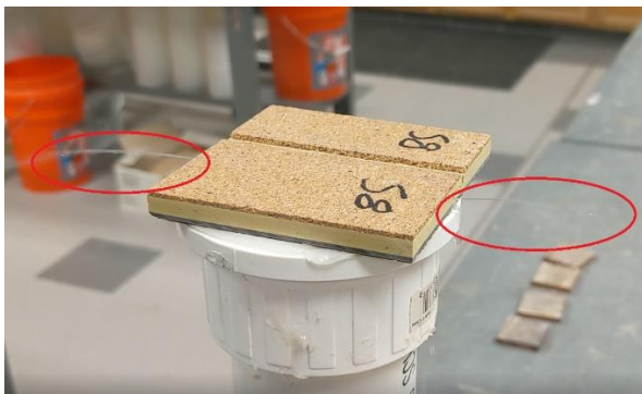
Figure 6.3.1: Water penetrating the seam and exiting from the edges
