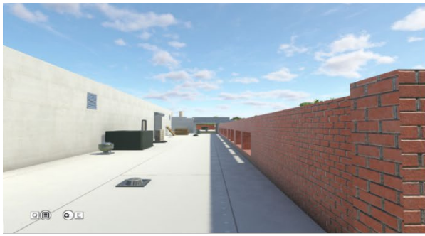
a. Roof parapet and rooftop equipment
