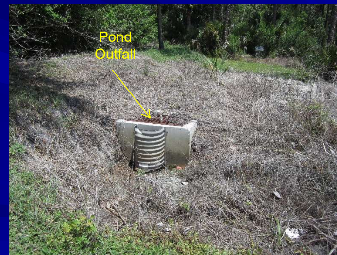
d. Pond 3 Outfall Structure
