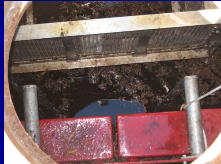
d. Baffle box unit following cleaning
