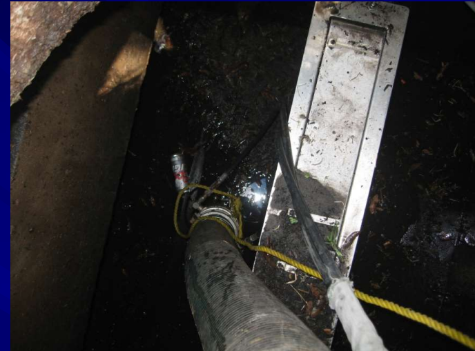
b. Standing water pumped from bottom chambers
