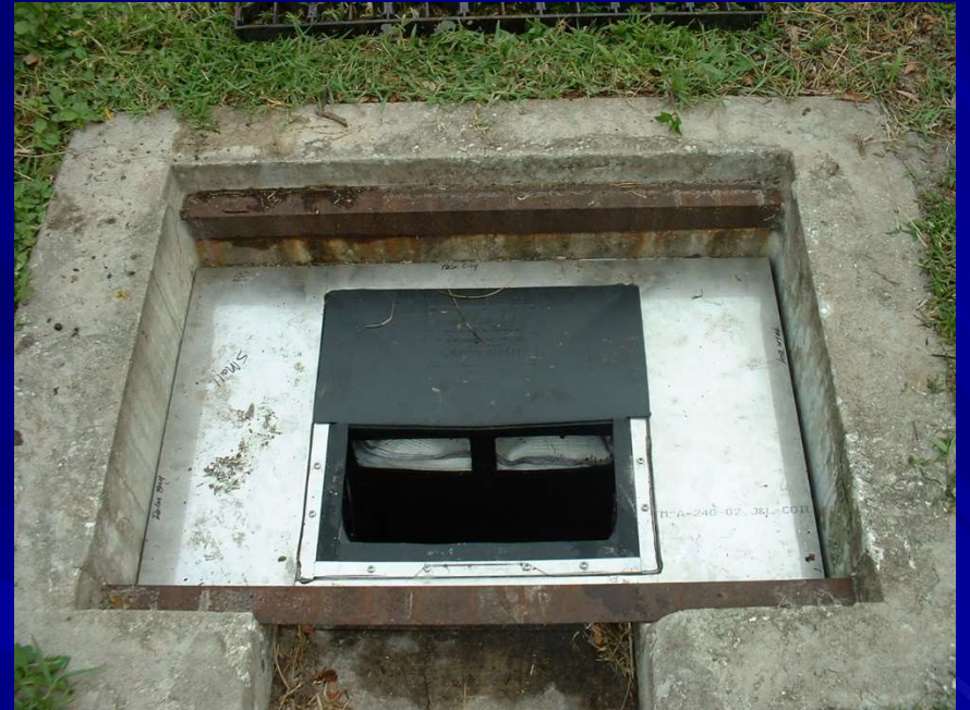
Hydro-Kleen Unit with Grate Removed
