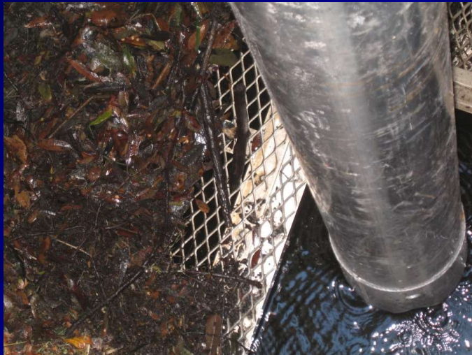
c. Solids vacuumed from chambers
