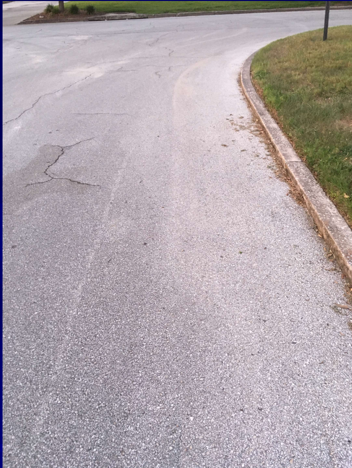
Mechanical sweepers grind up roadway solids and leave a homogenized "paste" on the roadway surface
