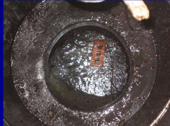
d. Sump area following cleaning
