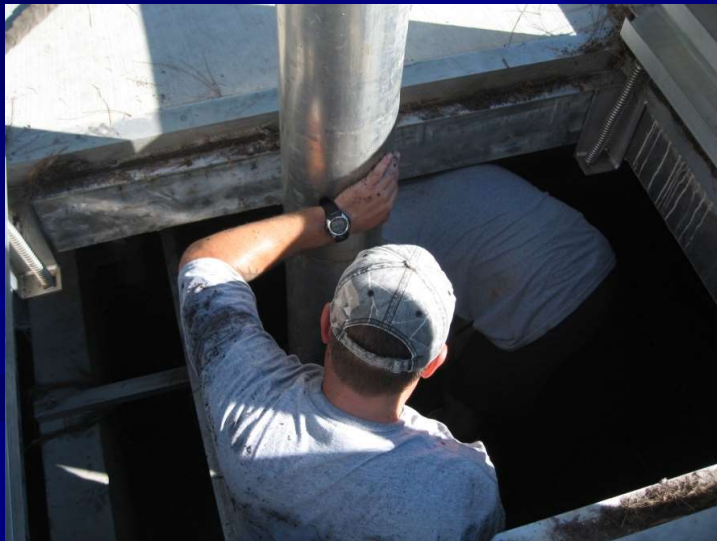
c. Solids removed from screen using Vector truck
