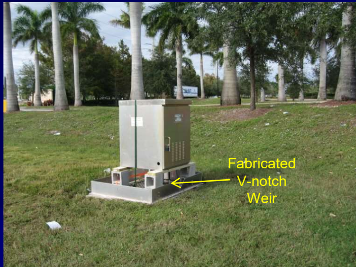
Site 2 – Overview of south pond
