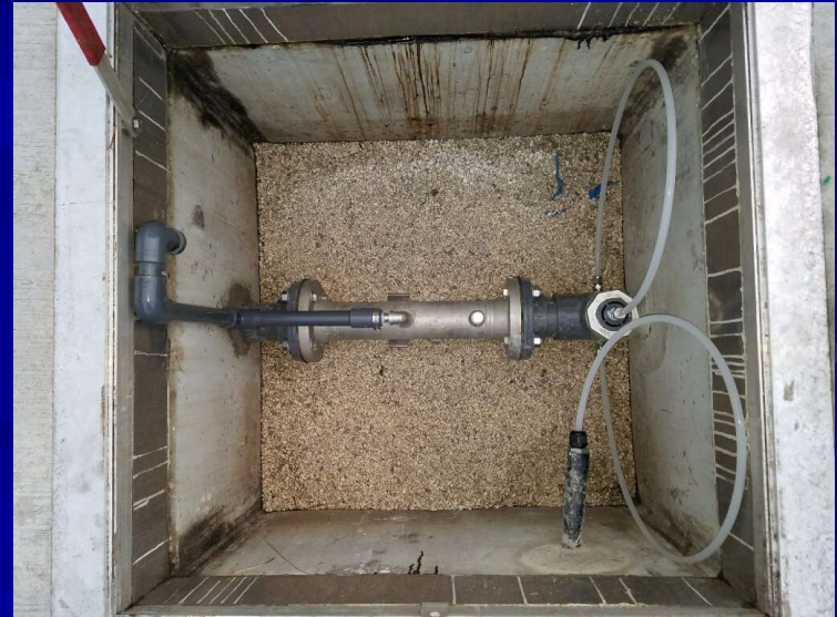
Venturi for Alum Addition
