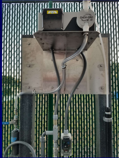
Alum metering pump
