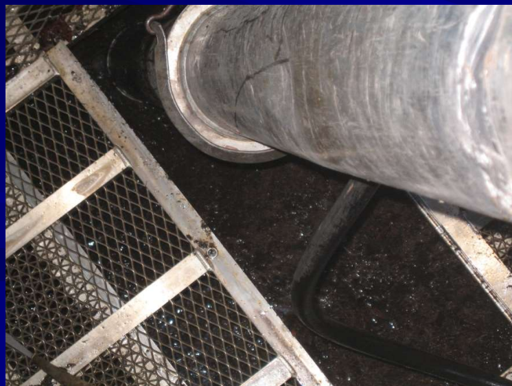
c. Solids removed using Vactor truck
