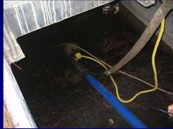
b. Standing water is pumped from the sump area
