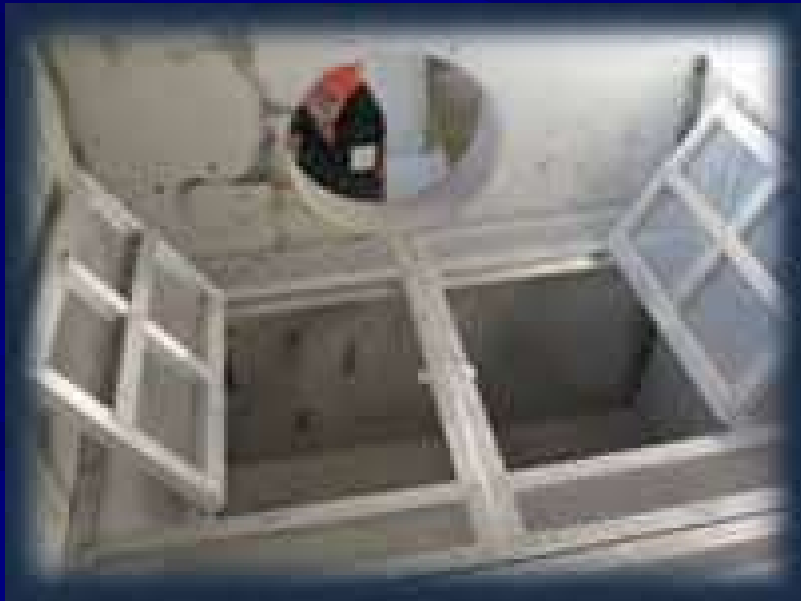
d. Bottom screens opened for cleaning
