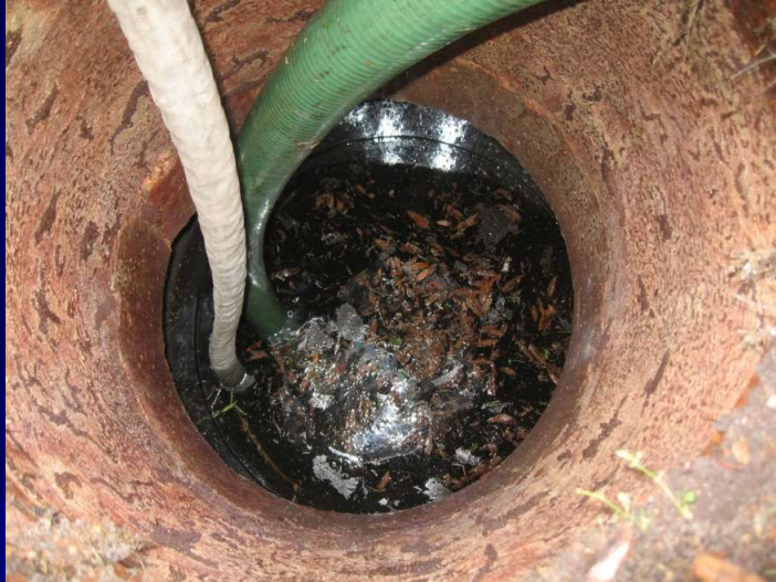
a. Interior of CDS unit prior to cleaning
