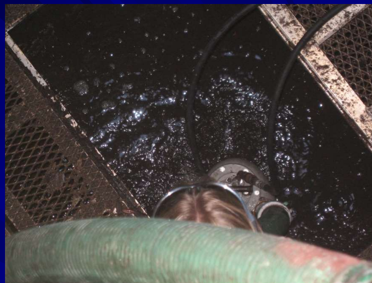
b. Water pumped from sump area
