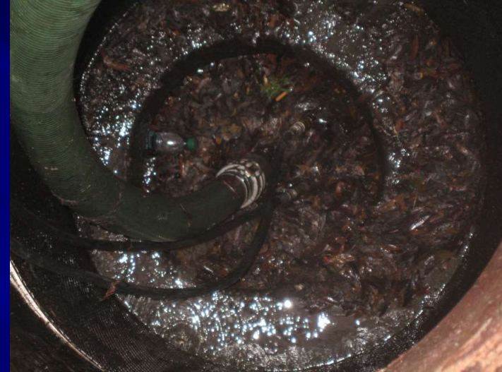
b. Standing water is pumped from the unit
