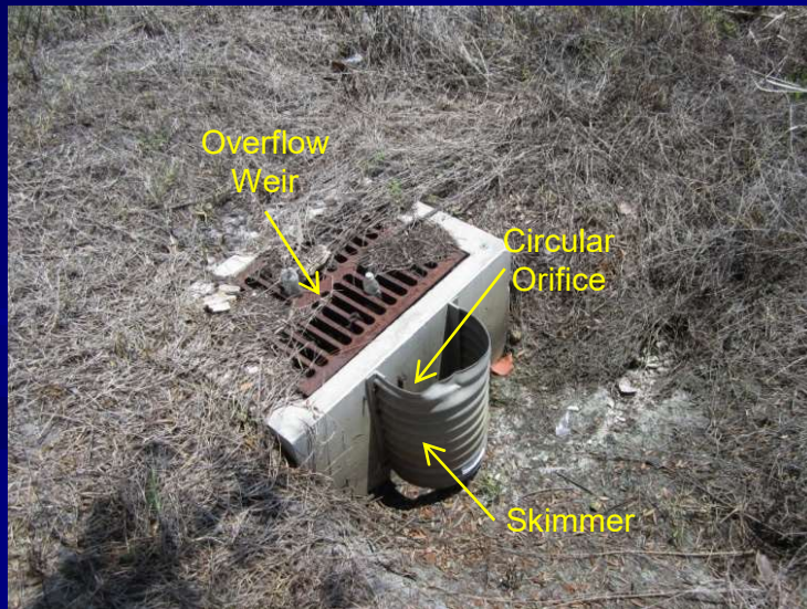
Site 5 – System Outfall to Canal
