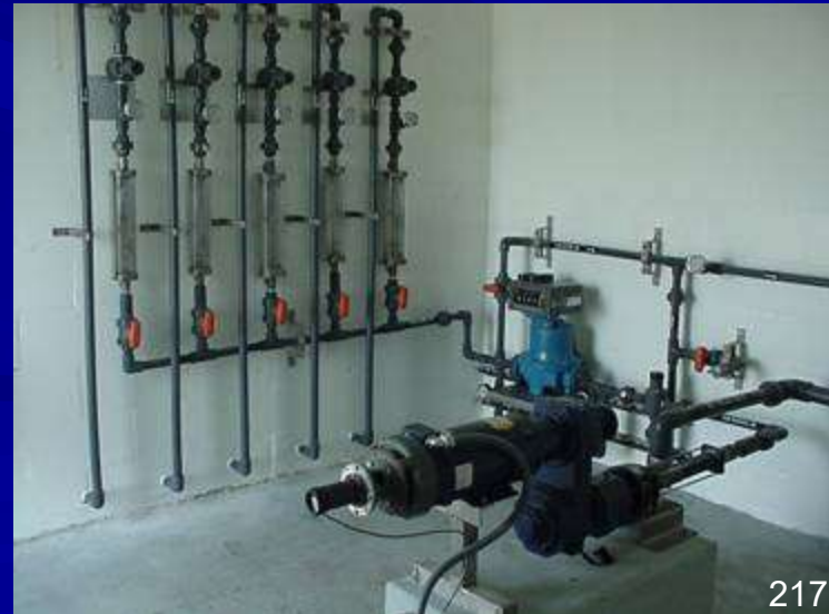
Alum Injection Equipment
