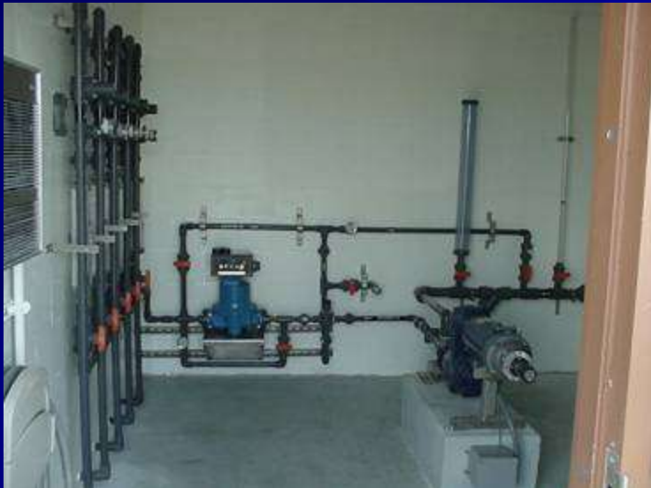
Alum Injection Equipment
