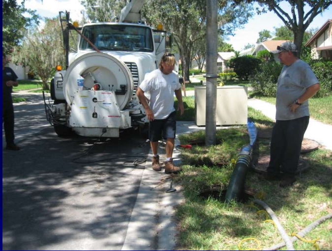
a. Cleanout operations
