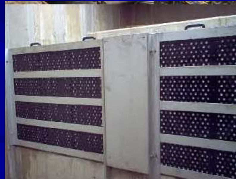
e. Outlet filter containing aluminum silicate
