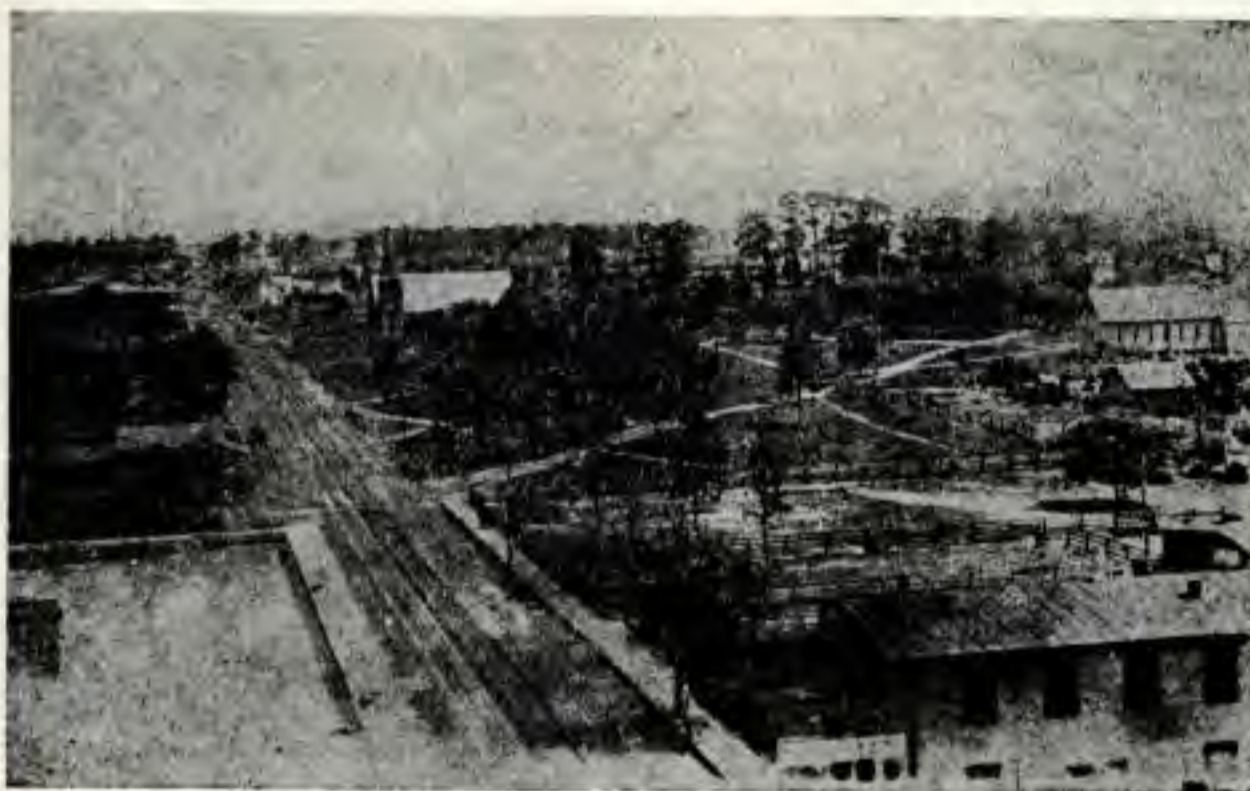
North Orange Avenue 1885, from East Central to Jefferson.
