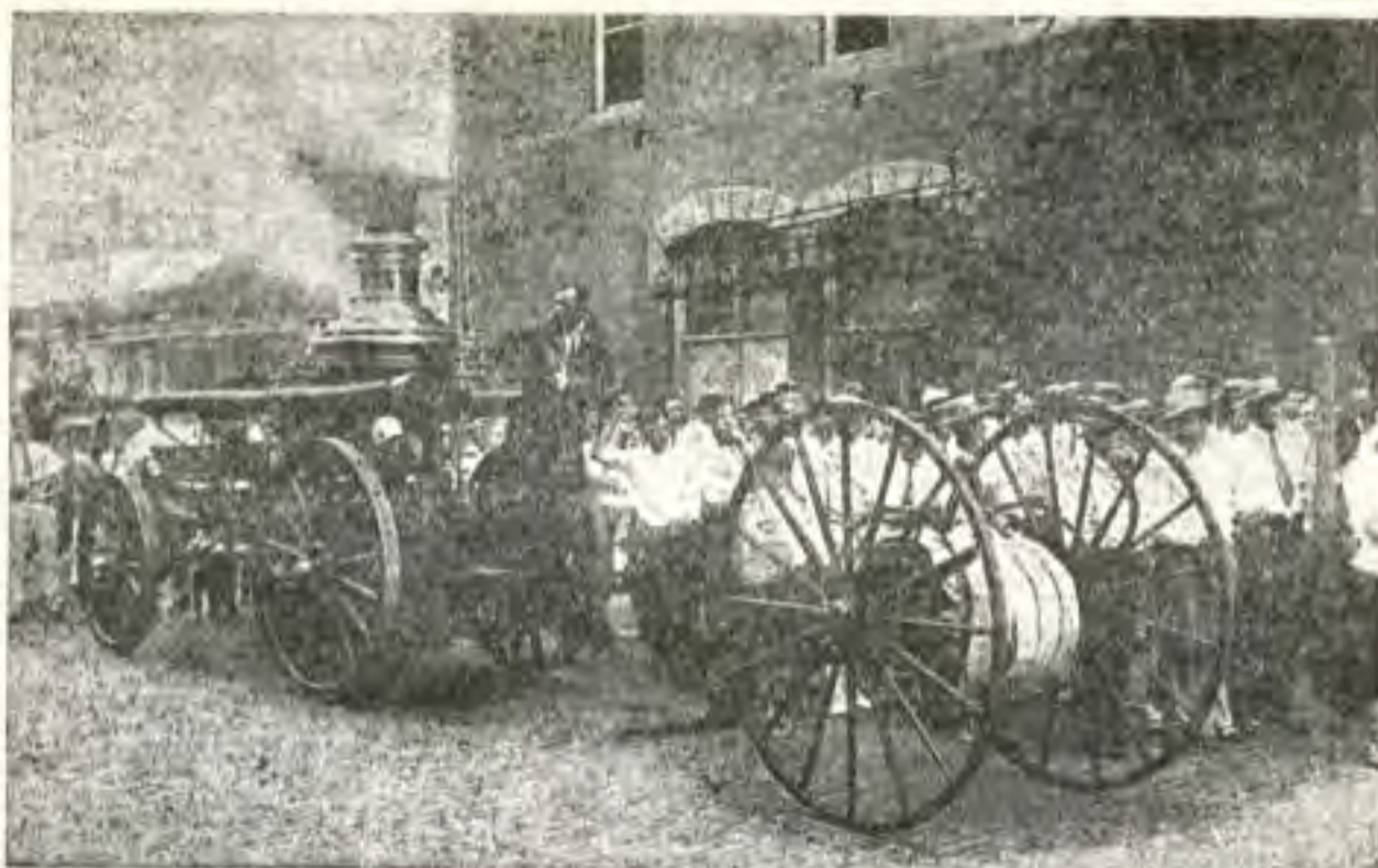
The Old Fire Engine, "Metropolitan" in 1912. Also an old hose reel.
