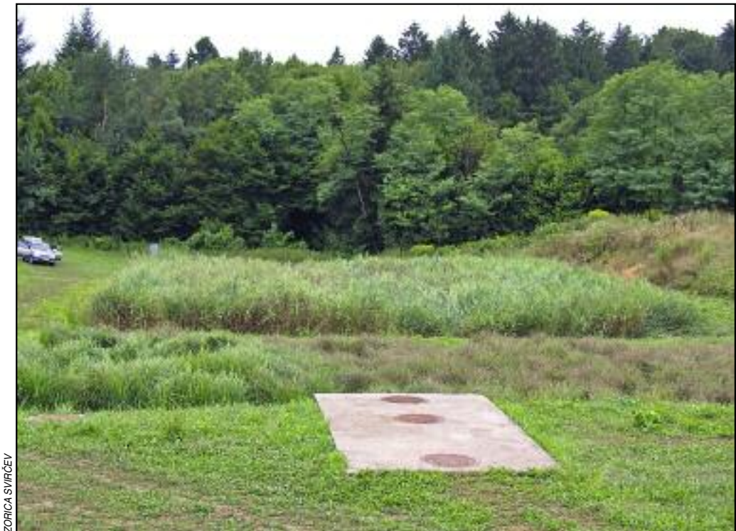
Figure 1: A constructed wetland for a domestic waste water treatment, Slovenia.
