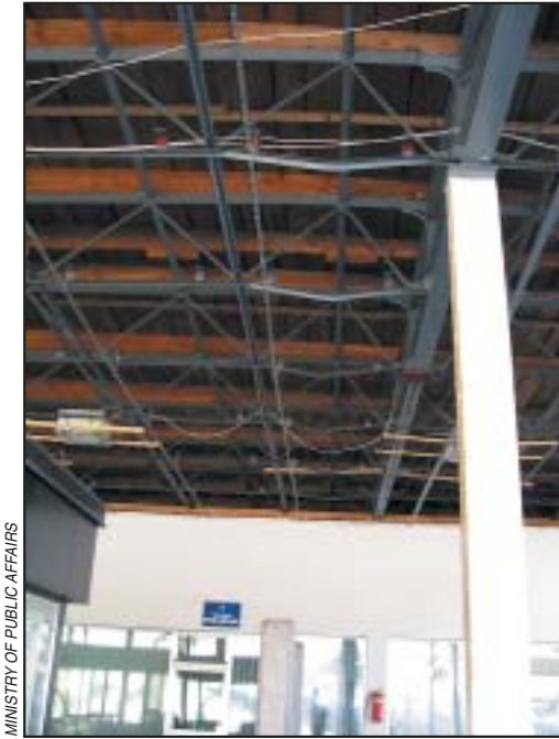
Figure 4: The deformation of the roof construction at the boarder crossing Rateče was so big that traffic underneath was stopped and reconstruction was necessary.
