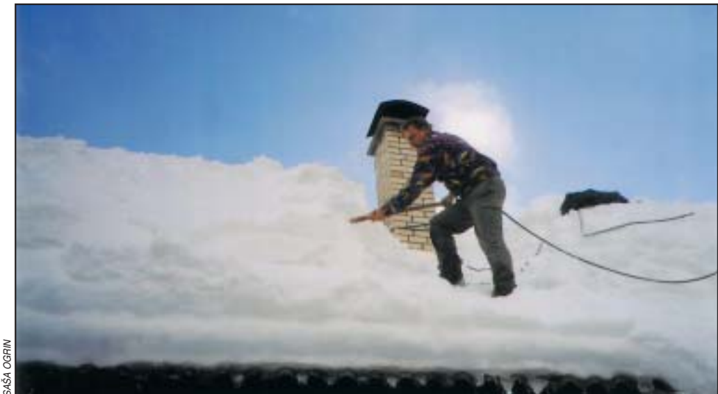
Figure 1: In the Upper Sava valley, some residents threw snow from roofs because of danger that snow would damage the roofs of buildings.
