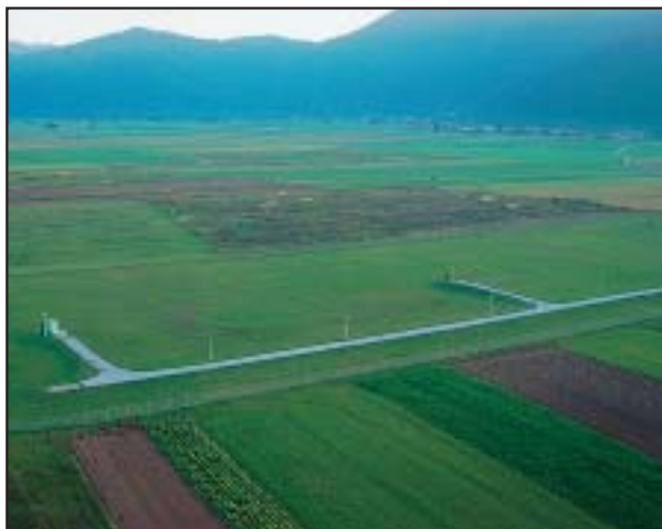
Brest water pumping station (photograph: Aleš Smrekar). Vodarna Brest (fotografija: Aleš Smrekar).
