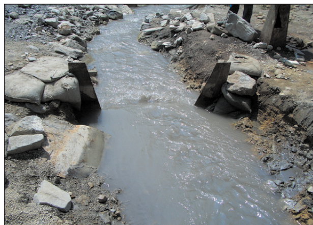
Fig. 3: Two photos of Zoumaling tunnel water inrush. Left: trapezoidal weir, located at tunnel entrance. Right: tunnel water inrush located at K47+350 (Photos: Q. Zhang).
