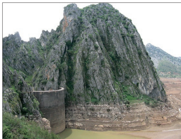
Fig. 12: Empty reservoir of Montejaque dam on Gaduares River in karst of southern Spain. Due to high leakage the reservoir was abandoned in the 1950s (Photo: Z. Stevanović).
