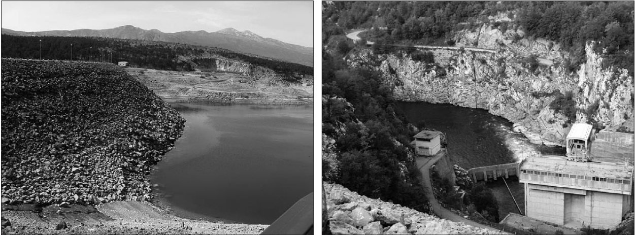
Fig. 7: The two dams in the Dinaric karst of Croatia: Cetina Reservoir and Peruća dam (left), Kruščica Lake and Sklope dam (right). Watertightness of Cetina is satisfactory (losses at the level of 1.5 % of average riverflow), while Kruščica has considerable water leakage ( \sim 1 \text{ m}^3/\text{s} ) (Photos: Z. Stevanović).
