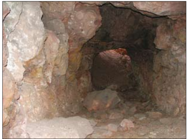
Fig. 9: Prospecting passage probably from the 1960s in the WID; view towards the entrance.
