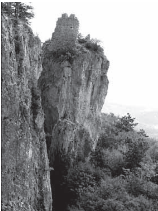
Fig. 2: Photo of the »Kraški rob wall« and the rock block whereon the castle of Črni kal is situated (Photo: M. Ribičič).
