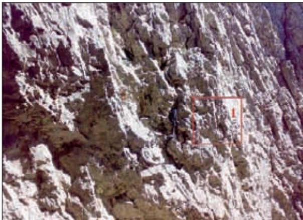
Fig. 7: Point 1 from the system (cloud) – Kraški rob wall (Photo: S. Konič).
