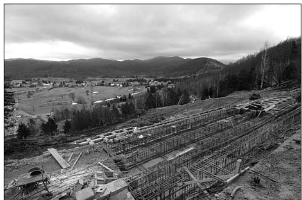
Fig. 13b: Constructing grid (Photo: M. Garašić).
