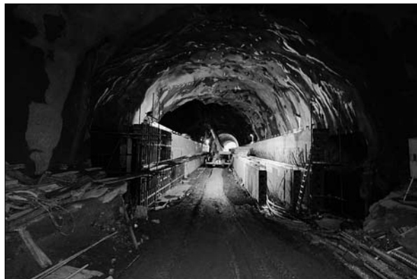
Fig. 11b: Bridge in tunnel (Photo: M. Garašić).
