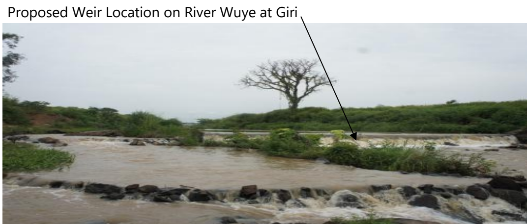
Figure 3: River Wuye at Giri , Abuja, Nigeria
