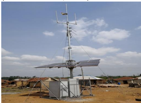
Figure 15: Rural Star 2.0 Small Cell in Nigeria (Source: Madeline et al., 2018)
